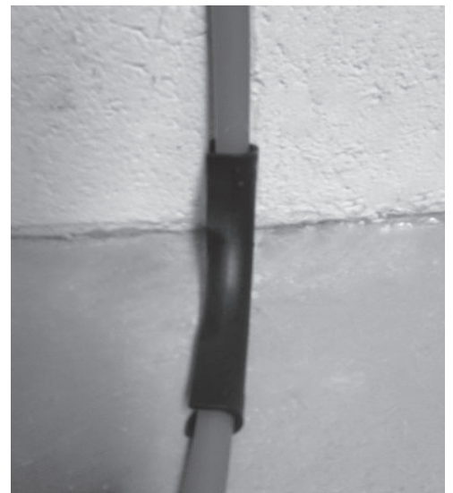
Use the Warmup Pipe Bend Support where it enters the floor.
